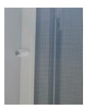
5. Once the screen has been hung in position secure the turn buttons in place to hold the fly screen panel closed.
