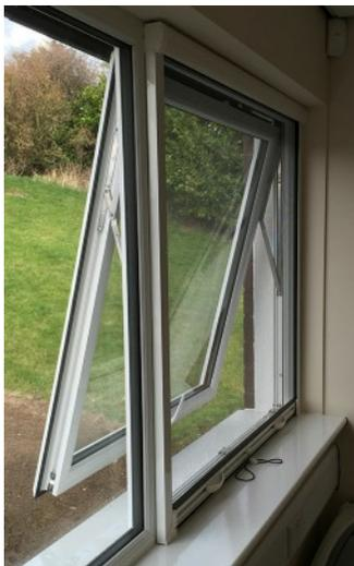
The screen is fixed directly to the face of the window frame.
