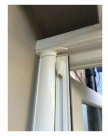
4. The top and bottom guides will now need to be installed onto the cassette and magnetic extrusion. Loosen the screws in the guide holders at the base and top of the extrusion and slide the holder up or down.
