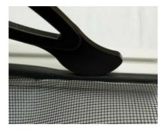
Once the mesh is held in place trim off any excess with a sharp Stanley knife, the mesh isn't supposed to be drum tight.
