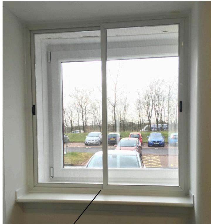
Make sure that the panels run on the edge of the frame and not inside the frame groove.
