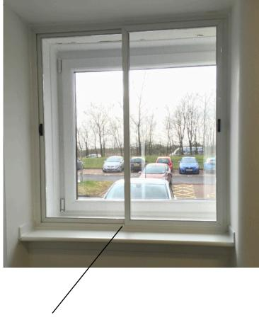
Make sure that the panels run on the edge of the frame and not inside the frame groove.
