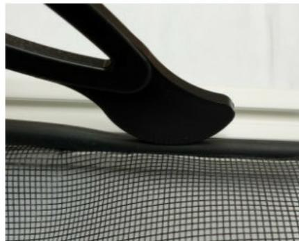
Once the mesh is held in place trim off any excess with a sharp Stanley knife, the mesh isn't supposed to be drum tight.
