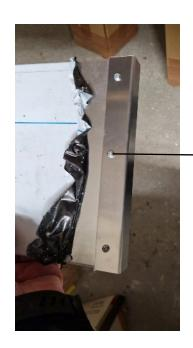
Attach the angled corner pieces to the canopy with either self tapping screws or rivets
