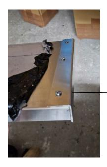
Attach the angled corner pieces to the canopy with either self tapping screws or rivets
