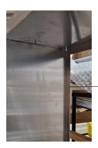
Once the canopy is assembled it can be fitted to your structure by drilling through the rear flange and then screwing it into position, ensuring that that you keep the canopy square.
